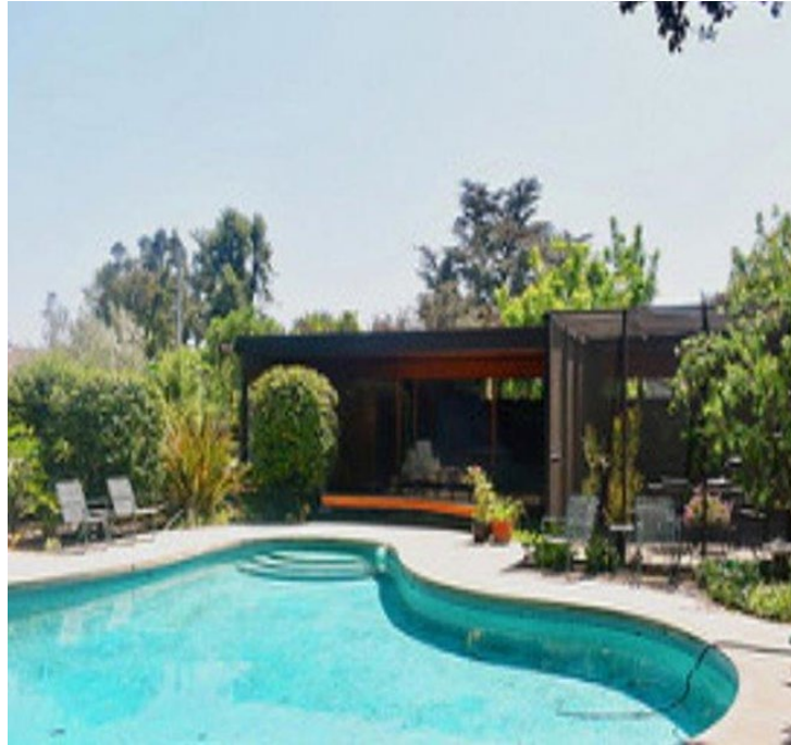
Figure 7 – The garden room is shown on the right tucked into the northeast corner of the Brod House
