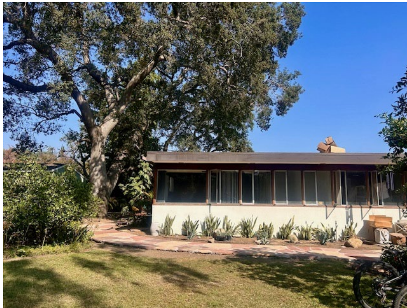
Figure 11 – West elevation of the Brod House, showing the master bedroom wing, rear garden, and oak trees on the property
