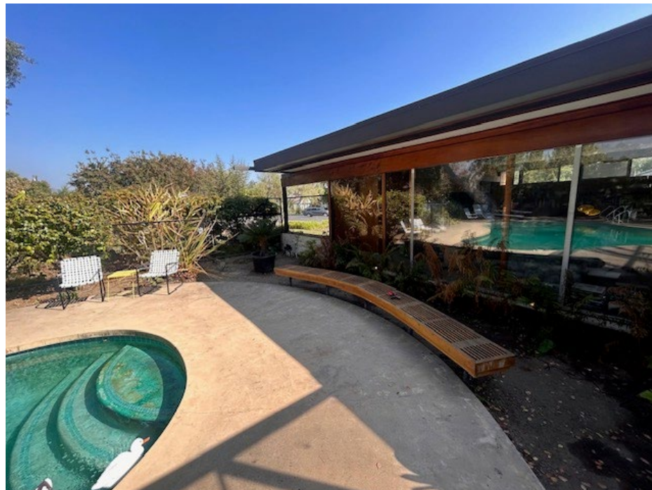
Figure 3 – The north elevation of the home that faces the swimming pool
