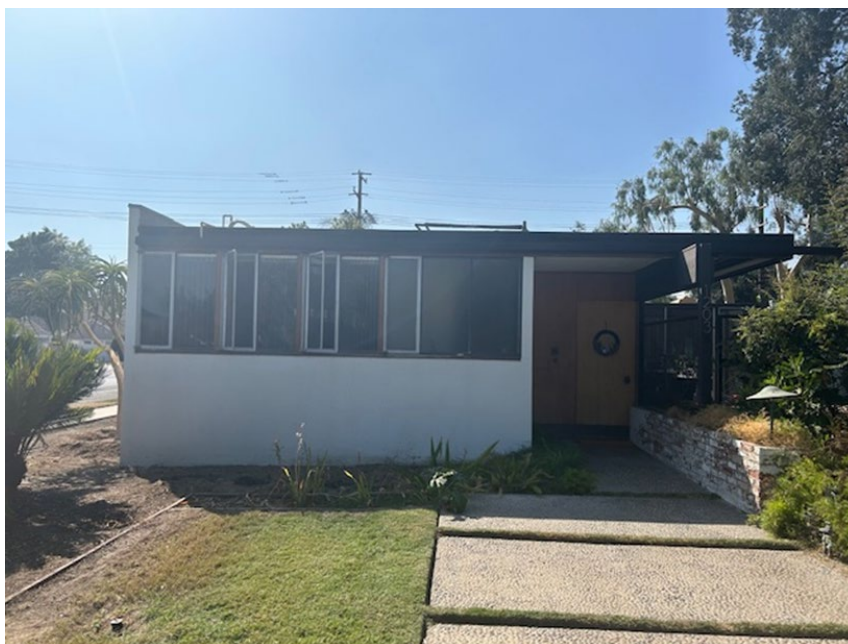
Figure 5 – The front elevation of the home. The “Factorlite” glass is the obscured glass on the 3 windowpanes furthest right.
