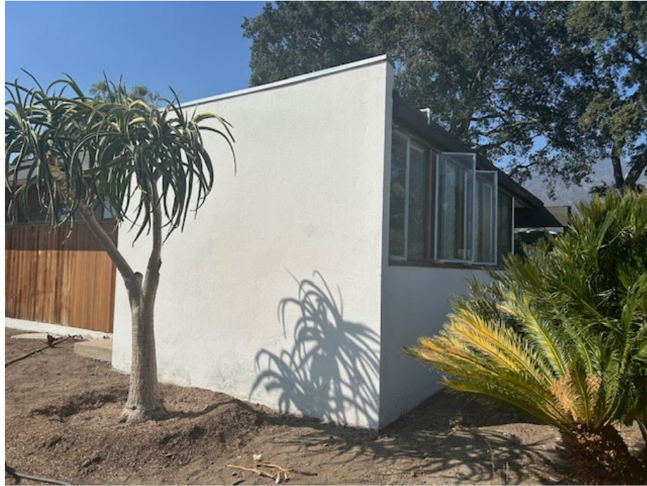
Figure 2 – Metal-capped stucco wall on the southeast corner of the house
