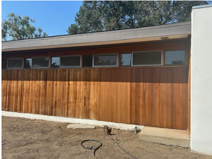
Figure 6 – The wood paneling along the south elevation of the house.
